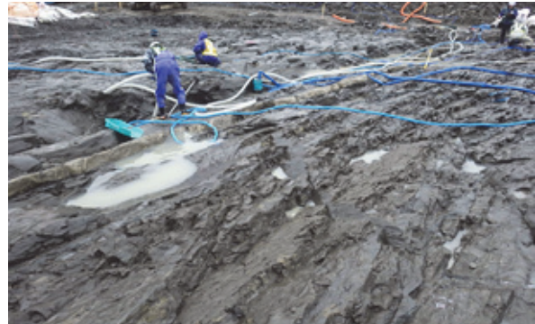
Figure 7. Unevenness of foundation rock
