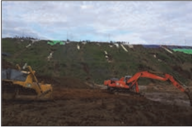
Figure 11. Dam Downstream Face Erosion
