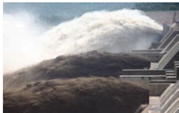
Figure 4. Water and sediment releasing process of density current in Xiaolangdi reservoir
