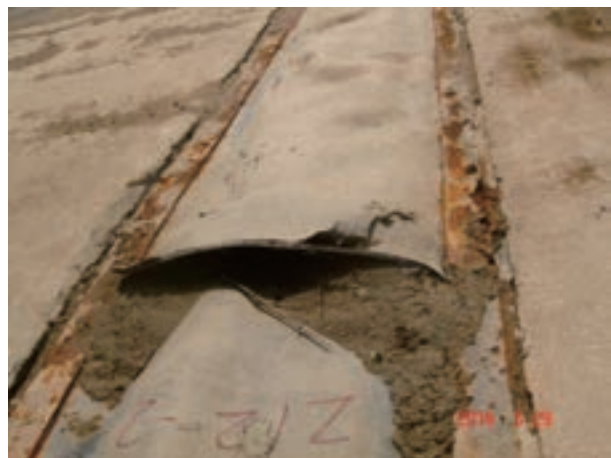
Figure1. Destruction of lapped joint of EPDM cover board
