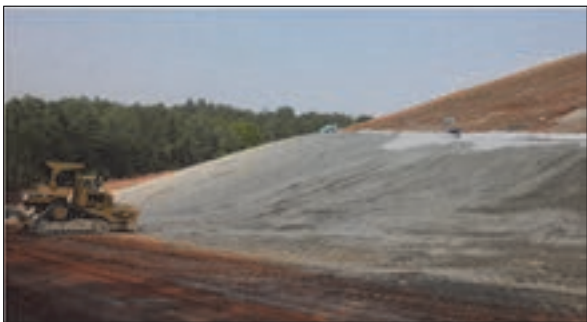
Figure 12. Filling the filter drain.
