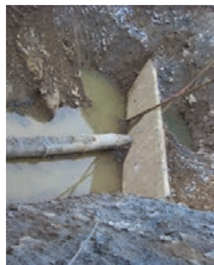
Figure 5. Photo of connection of the seepage measuring house and the collecting wall (after excavation for replacement)
