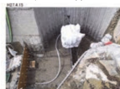
3rd lift before concrete placing (EL194.75)
