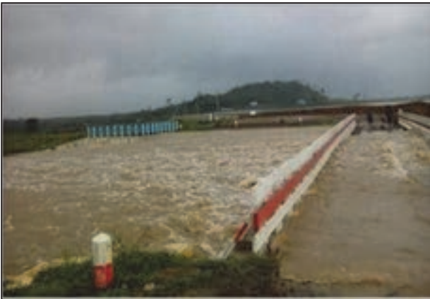
Figure 7. Submergence of Spillway-bridge
