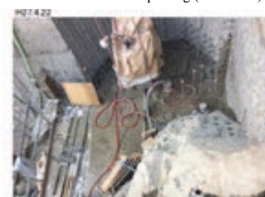
4th lift after concrete placing (EL196.25)
