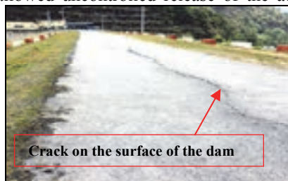
Figure 1. Crack on the crest of Kulekhani dam damage of penstock of Bhotekoshi Hydropower Project (courtesy of Neupane Hara Raj and Bikram Sthapit).
