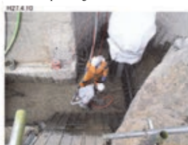
2nd lift before concrete placing (EL194.0)
