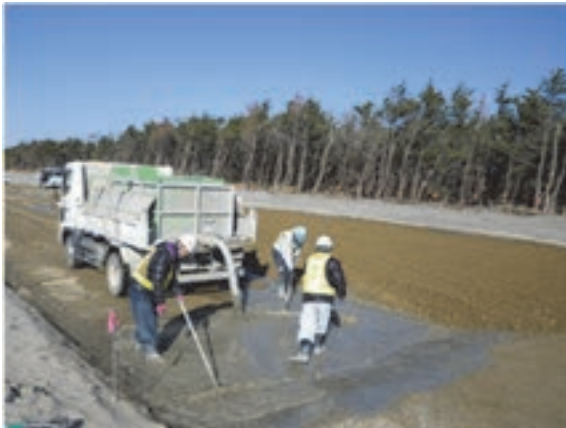
[1] Applying cement paste
