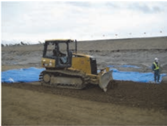
[3] Spreading of CSG
