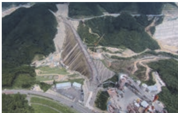
Figure 1. View of dam body placement (View of placement work on July 31, 2015, EL401.5m, 88 lifts)
