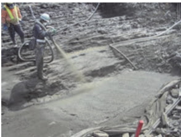
Figure 16. Shotcrete with mortar
