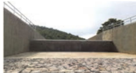
Figure 10. Storage capacity increase by building a weir at spillway
