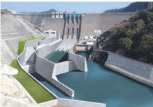
Figure 1. Conceptual drawing of completed redevelopment work (White colored parts are redeveloped.)
