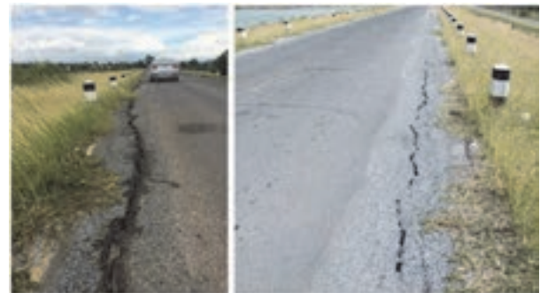
Figure 2. Longitudinal cracks were found on dam crest. (Office of Water Management and Hydrology, 2013)
