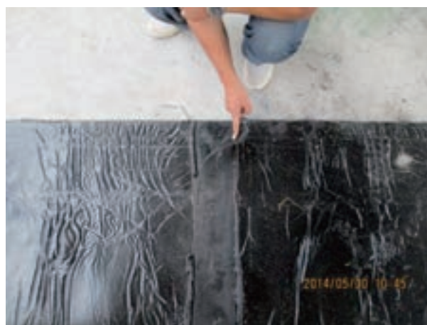
Figure.9 Butt joint of EPDM cover boards by vulcanization
