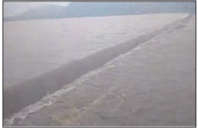
Figure 9. Dam Overtopping
