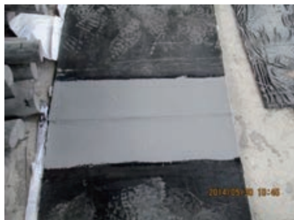
Figure.10 Lapped joint of EPDM cover boards with polyurea with PET nonwoven substrates coating
