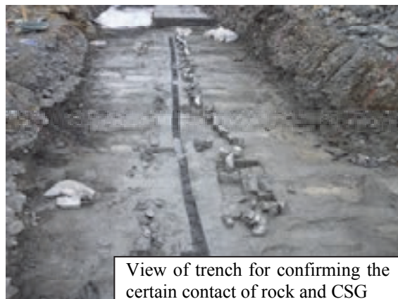
Figure 14. Filling of CSG to concave parts of foundation rock
