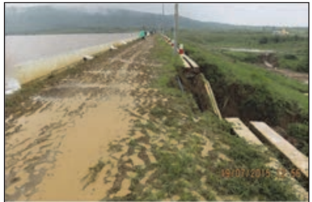
Figure 10. Dam Crest Erosion
