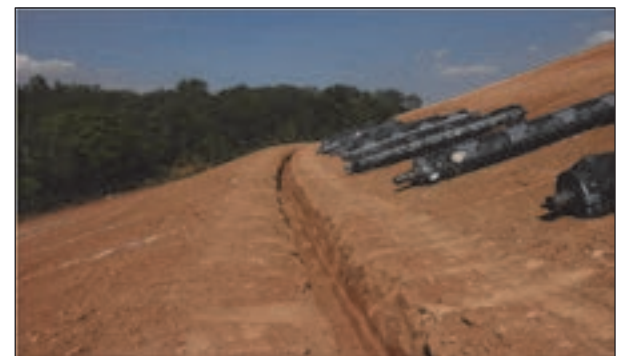
Figure 10. The anchored trench
