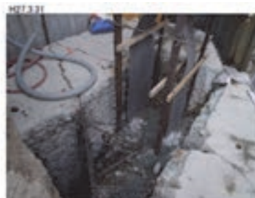
Water-stop setting in the rock foundation
