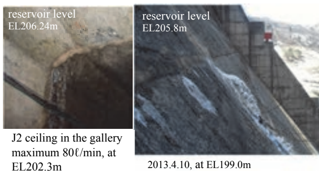
Figure 11. Water leakage situation through the J2 joint
