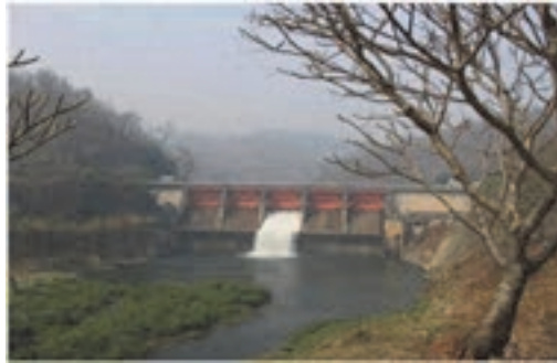
Figure 11. A large-scale dam uses watergates to control water at spillway
