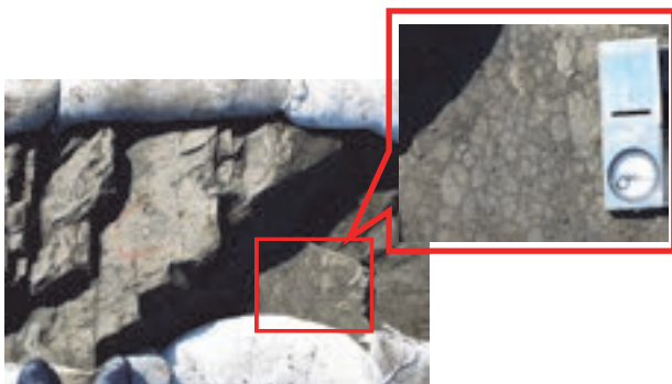
Figure 10. State of foundation rock (after 1-hour exposure)
