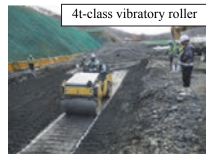
Figure 13. Execution of rock contact part
