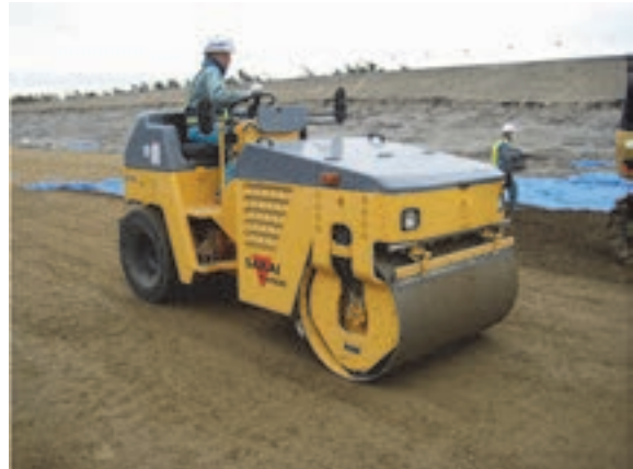
[4] Roller compaction
