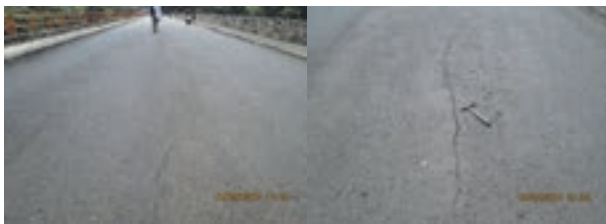
Figure 1. The longitudinal cracks on the dam crest with 0.3 to 0.5 cm width
