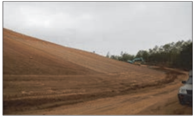
Figure 13. Filling the top soil layer
