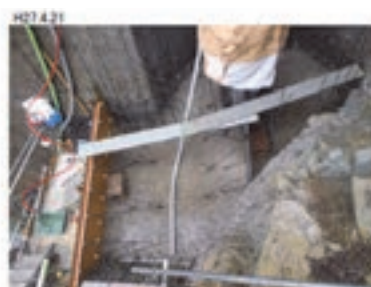
4th lift before concrete placing (EL195.5)
