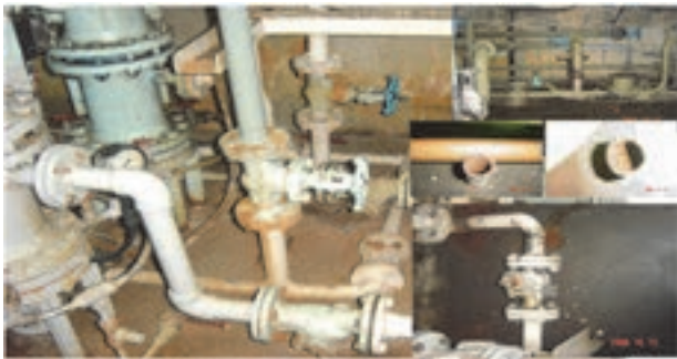
Figure 4. The rotten and corrosion of HEPP equipment and infrastructure
