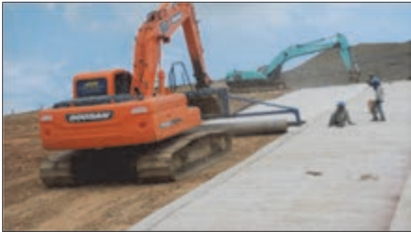
Figure 11. The GCL with textured HDPE installation procedure
